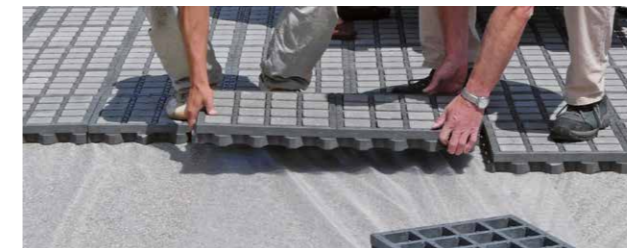
For a more efficient procedure, the TTE® elements can also be laid pre-filled as TTE® directPAVE. Mechanical installation is also possible in this way.
